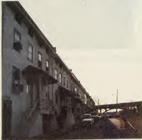
Fig. 112 Row of workers' housing on the edge of the French Creek Basin. Photograph by the author, 1995.
